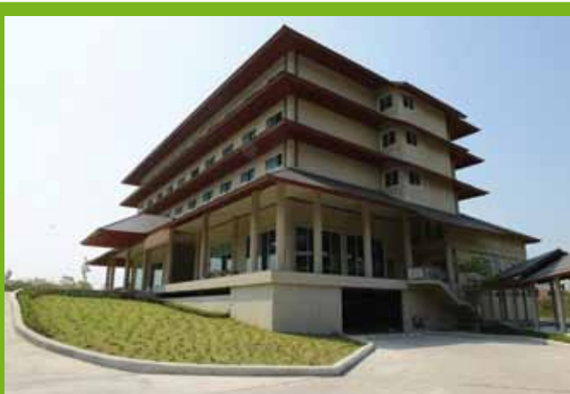
KASIKORNTHAI Learning Center located in Bang Pakong District, a green building concept certified by LEED
