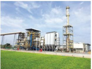
wood into Refuse Derived Fuel (RDF) and supply it to the power plant for producing electricity of 56,888,000 kilowatts-hour per year.
