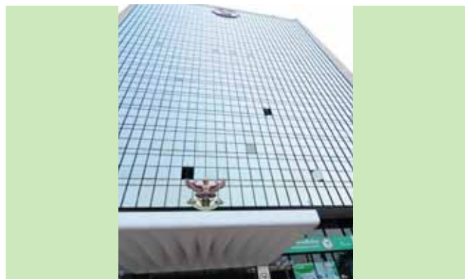
The Phahon Yothin Main Branch under renovation, including its piping work system and floor plans, in an attempt to make the old building “green” in accordance with international standards.
